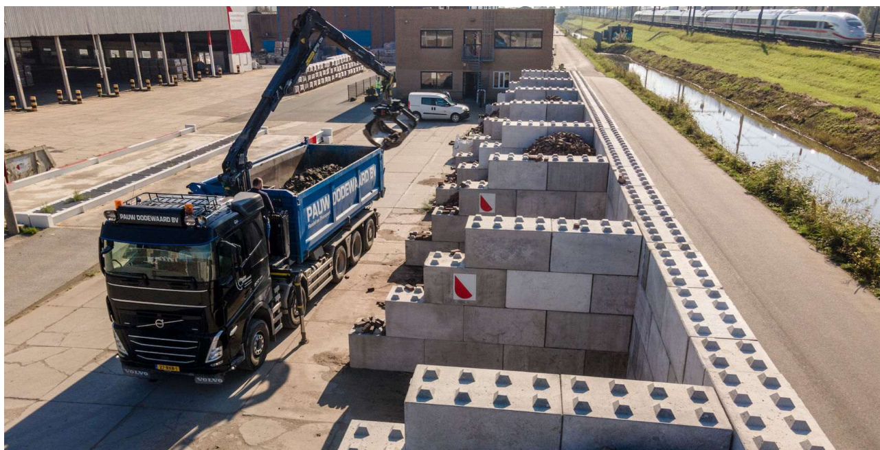
Prefabricated stackable concrete blocks and truck at Trechterweide. City of Utrecht, 2025. © City of Utrecht
